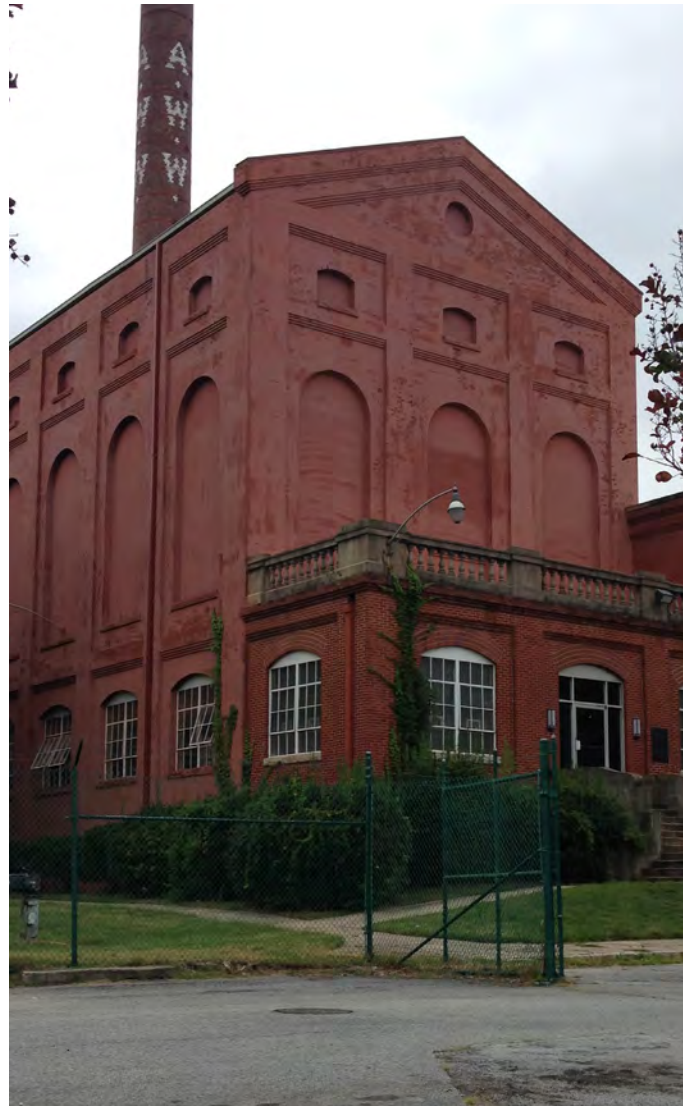
Hemphill Avenue Pump Station
