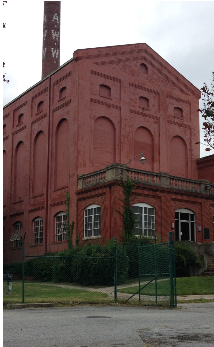
Hemphill Avenue Pump Station
