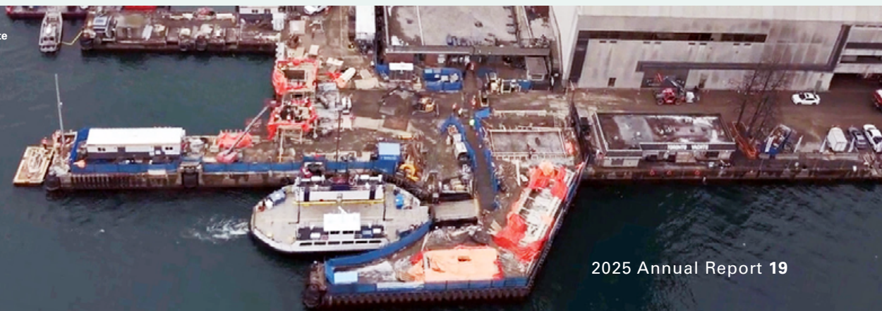
Jack Layton Ferry Terminal Construction Site
