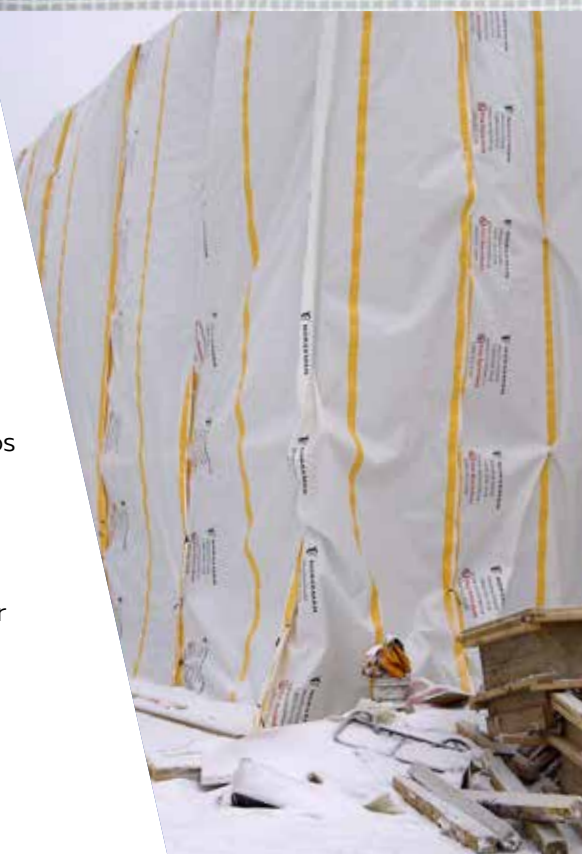
Manufactured with scrim-reinforced polyethylene material.
